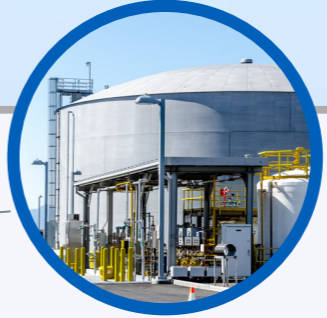
Silicon Valley Advanced Water Purification Center
