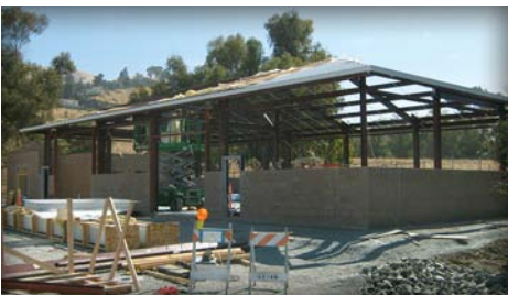
Penitencia Water Treatment Plant Maintenance Building
