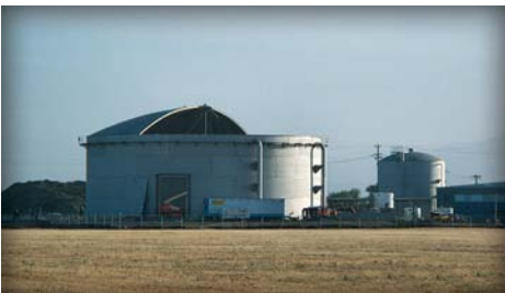
Silicon Valley Advanced Water Purification Center
