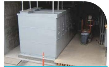
**New Switchgear at RWTP:** This is new state-of-the-art 12.47kV switchgear with enhanced personnel safety features, operating capabilities, and capacity for future loads.
