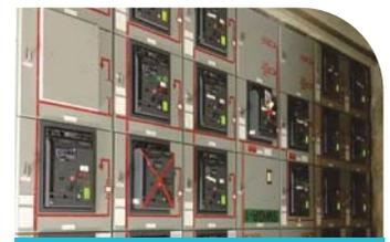
**New Switchgear at RWTP:** This is new state-of-the-art 480V switchgear with enhanced personnel safety features, operating capabilities, and capacity for future loads.
