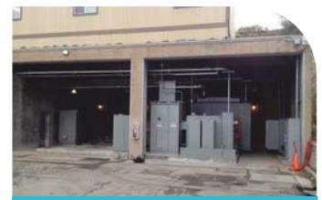
**New Transformers:** These two new transformers were installed during second shutdown and currently providing electrical power to RWTP, the second set of redundant transformers will be installed during third shutdown which is scheduled for March 12, 2012.
