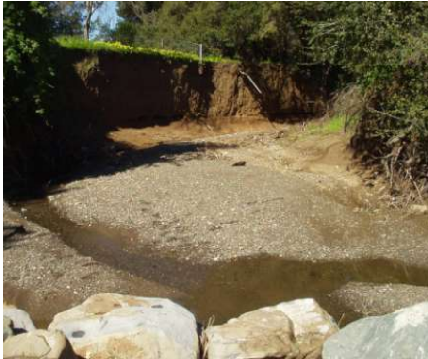
Figure 8-3. Example of Bank Erosion in Thompson Creek
