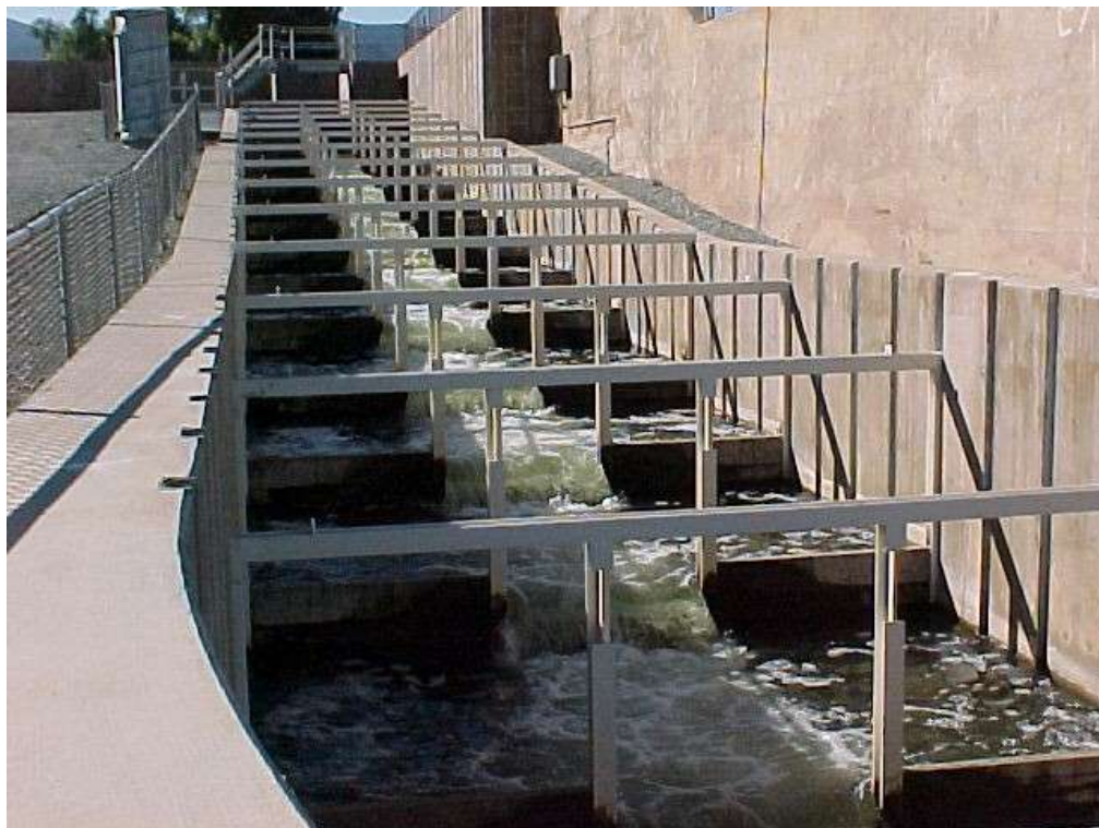
Figure 6-7. Pool and Weir Fishway at Alamitos Drop Structure
