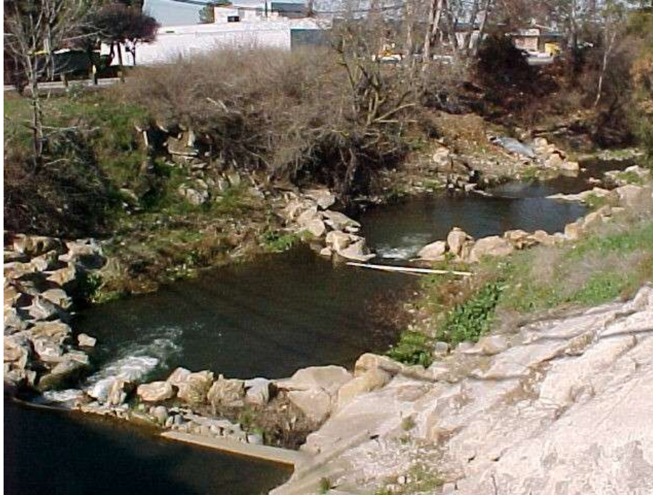
Figure 6-6. Hillsdale Rock Weir Fish Passage Improvement
