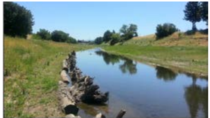
An example of a wood debris jam structure that will be installed at the Reach 12 location.
