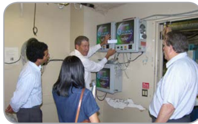
Ozone laundry system being installed
