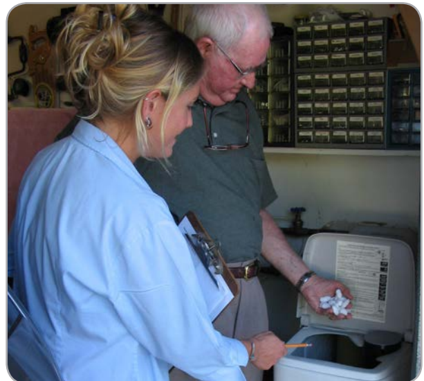
District staff inspects water softener
