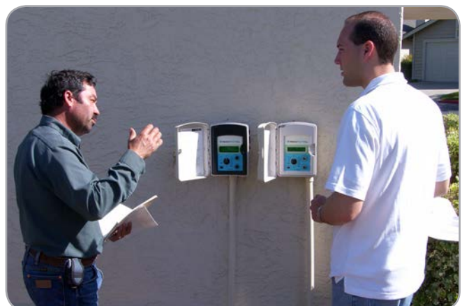
Weather-based irrigation controller installed at a Silicon Valley company.
