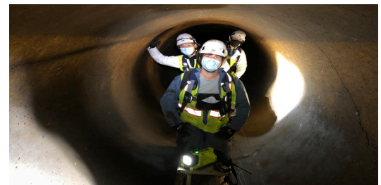
Crews working on the 10-Year Pipeline Inspection and Rehabilitation.
