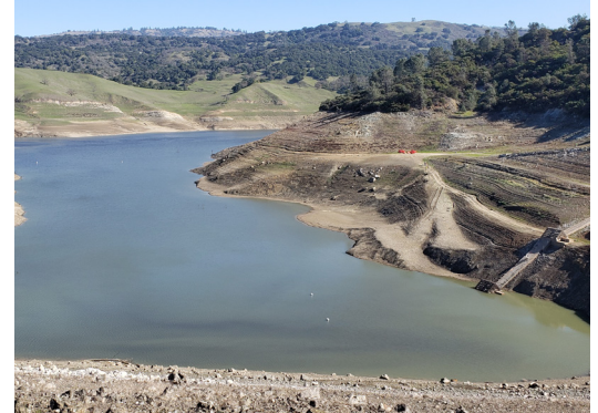
Site of the Anderson Seismic Retrofit and FERC Compliance Projects.
