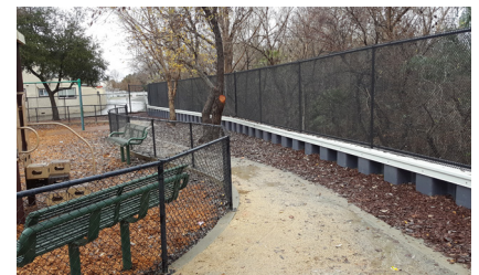
Coyote Creek Flood Protection Project.
