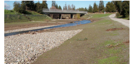
Site of the Upper Guadalupe River Reach 6 Gravel Augmentation Project.
