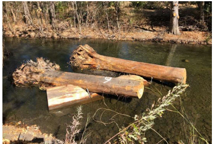
Installed Large Woody Debris.
