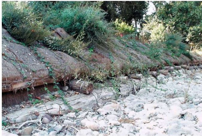
Site of completed erosion repair.
