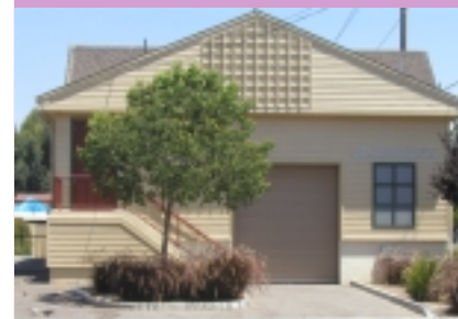
Improvements to several system pump stations was part of the district's agreement with South bay Recycled Water Program. This pump station, located near San Jose State University, was designed to reflect the architecture in the area.
