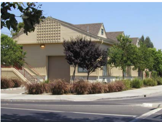
Part of the District's agreement with the South Bay Water Recycling Program includes improvements to several system pump stations, such as this one near San Jose State University.
