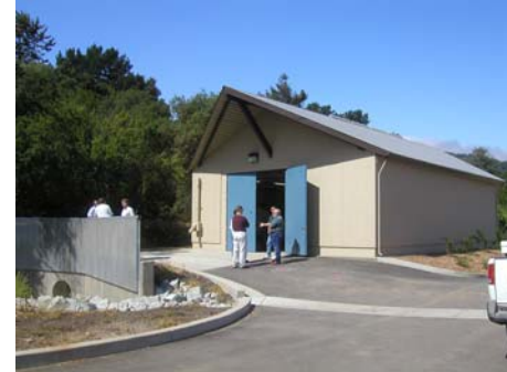
As part of the South County Recycled Water upgrade, the District constructed this new booster pump station at Christmas Hill Ranch Park.
