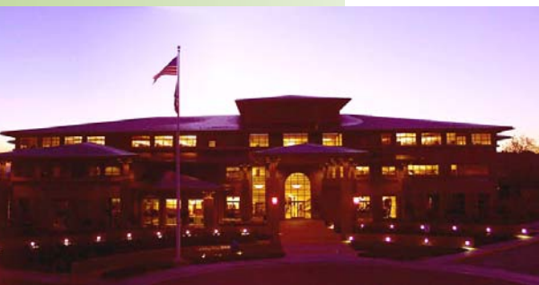
Santa Clara Valley Water District offices.
