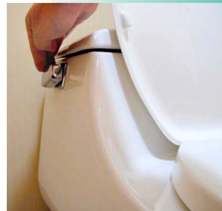
The District installed over 20,000 residential ULFTs during fiscal year 2002.
