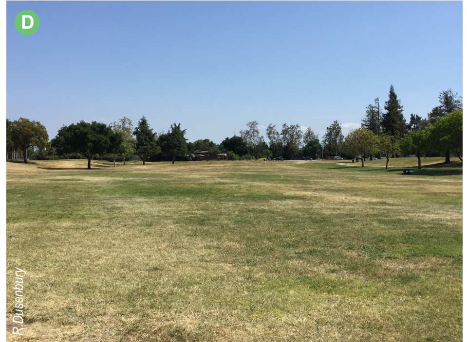
(D) With Minimal Earthwork, a Natural Basin at the West End of the Park will Provide Flood Control
