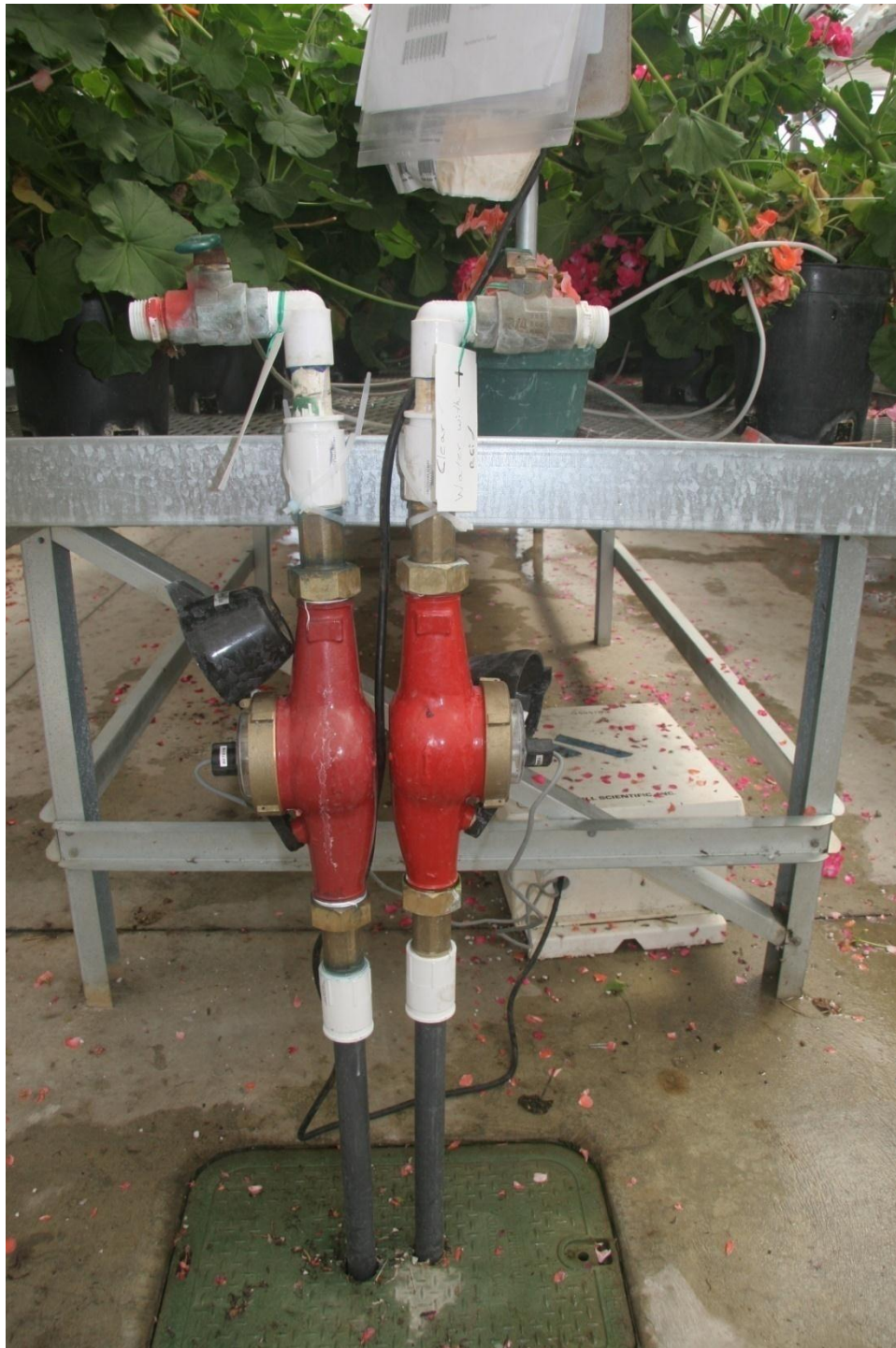
Greenhouse Flow meter installation
