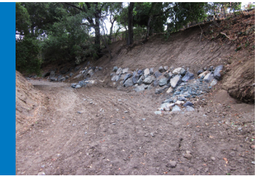
After Erosion Repair
