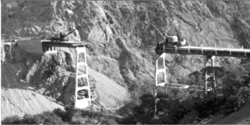
Construction at Anderson Reservoir, 1951
