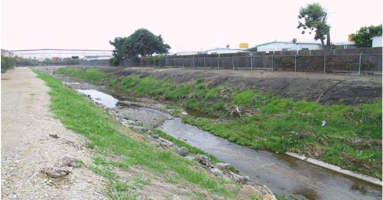
Before – Canos Creek u/s Hillsdale
