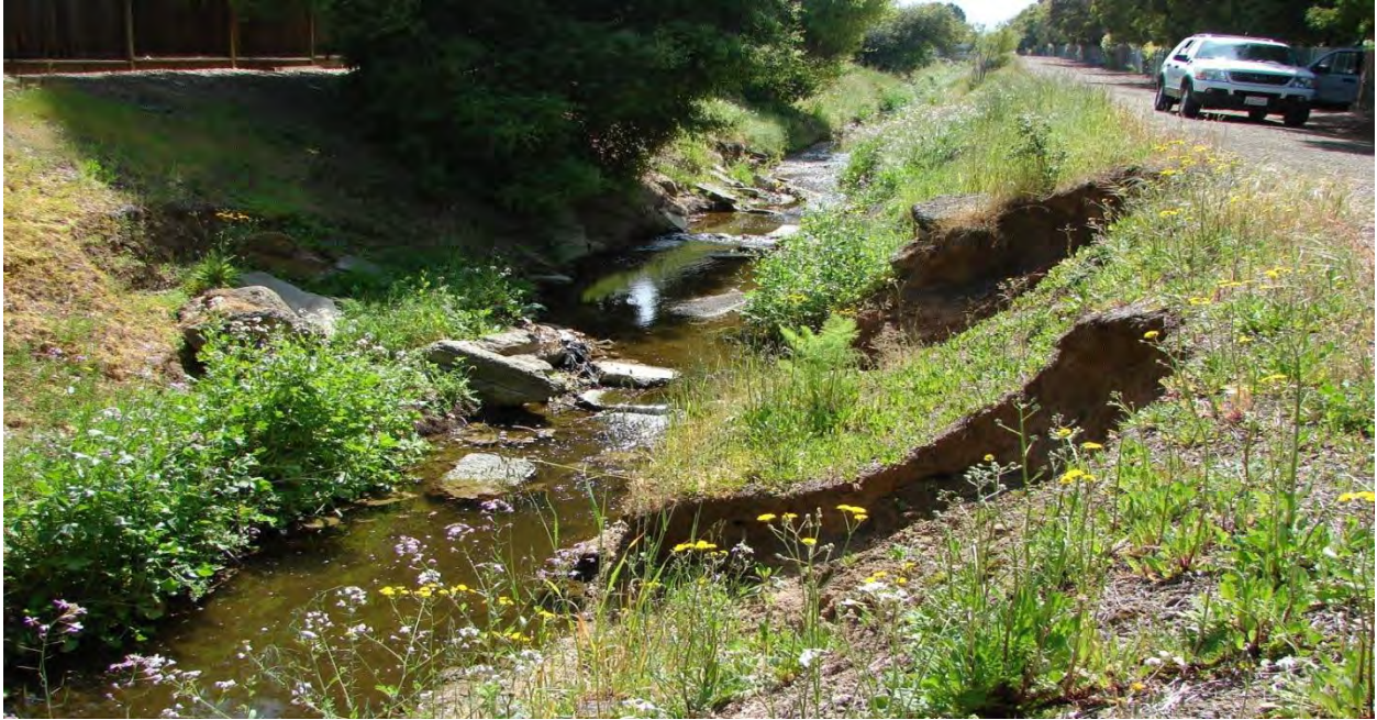
Before – Regnart Creek d/s Pacifica
