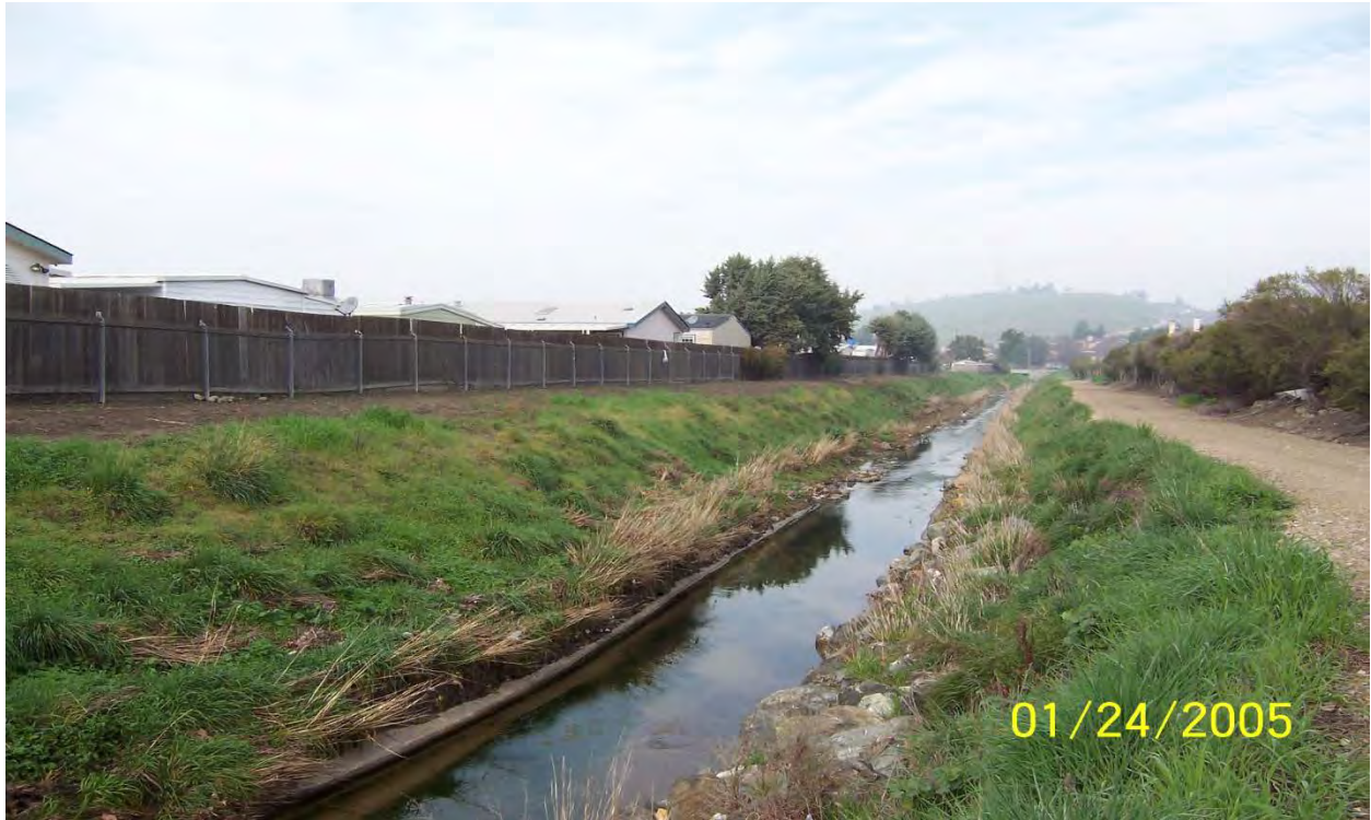
Before – Canos Creek u/s Hillsdale
