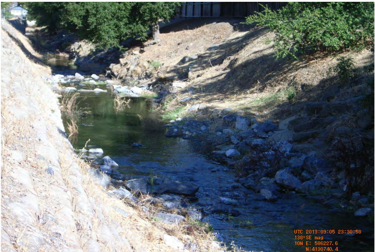
After – Regnart Creek d/s Pacifica
