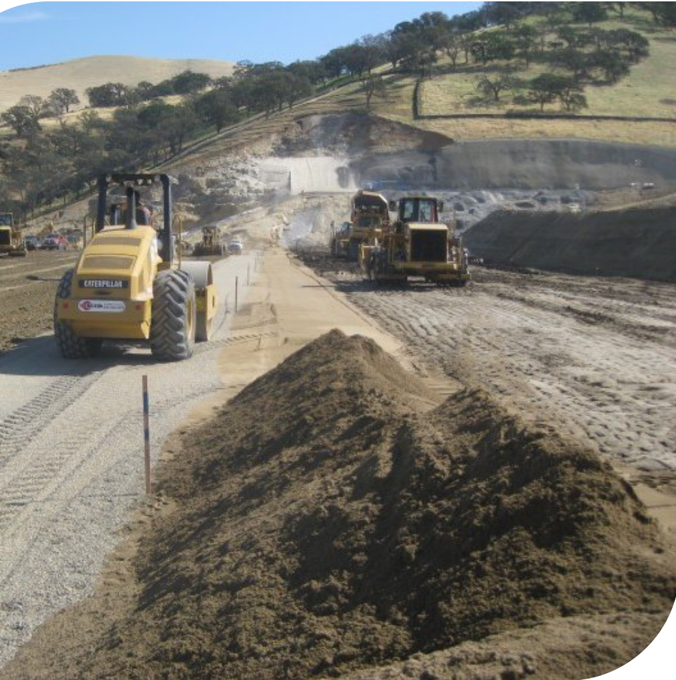
Pictured above: Earthfill Dam Construction in Bay Area
