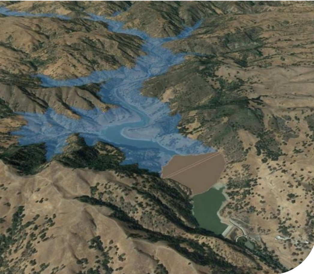
Pictured above: Earthfill Dam at Downstream Dam Site with 140,000 acre-feet Expanded Reservoir
