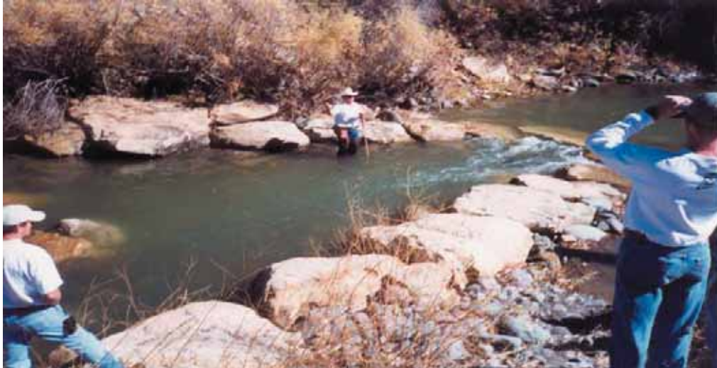
Photograph 1: Rock Cross Vane Structure:
