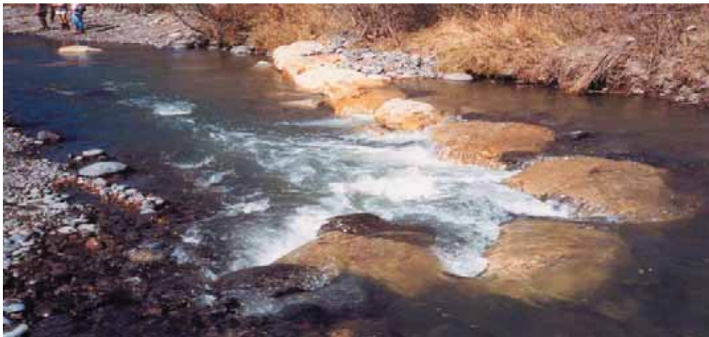
Photograph 2: Rock J-Hook Structure:
