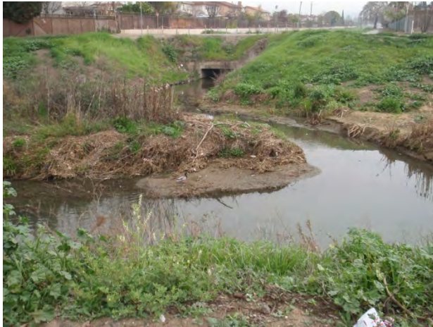
Figure 2-8. Confluence point of Norwood Creek and Lower Silver Creek, looking toward the east bank
