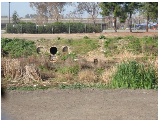
Figure 2-10. Outfalls on the west bank of Lower Silver Creek
