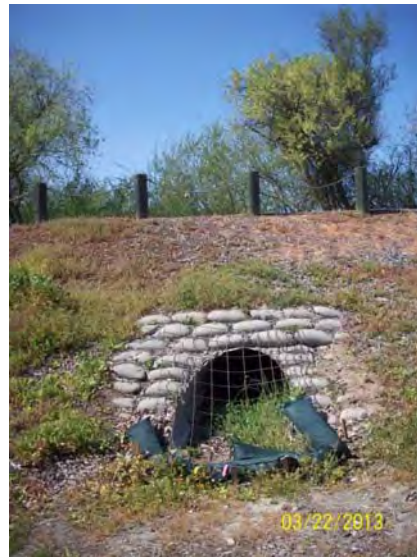
Figure 2-4. Outfall for Big Meadow Drainage into Lower Silver Creek close to Cunningham Avenue
