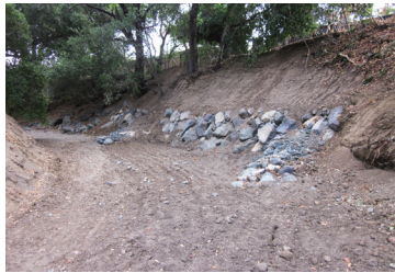
After Erosion Repair
