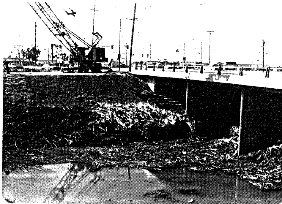
Trees in the bottom of many creeks caused major blockages to flow and required removal. Shown here is the trunk of a tree removed from San Francisquito Creek downstream of Chaucer Avenue.
