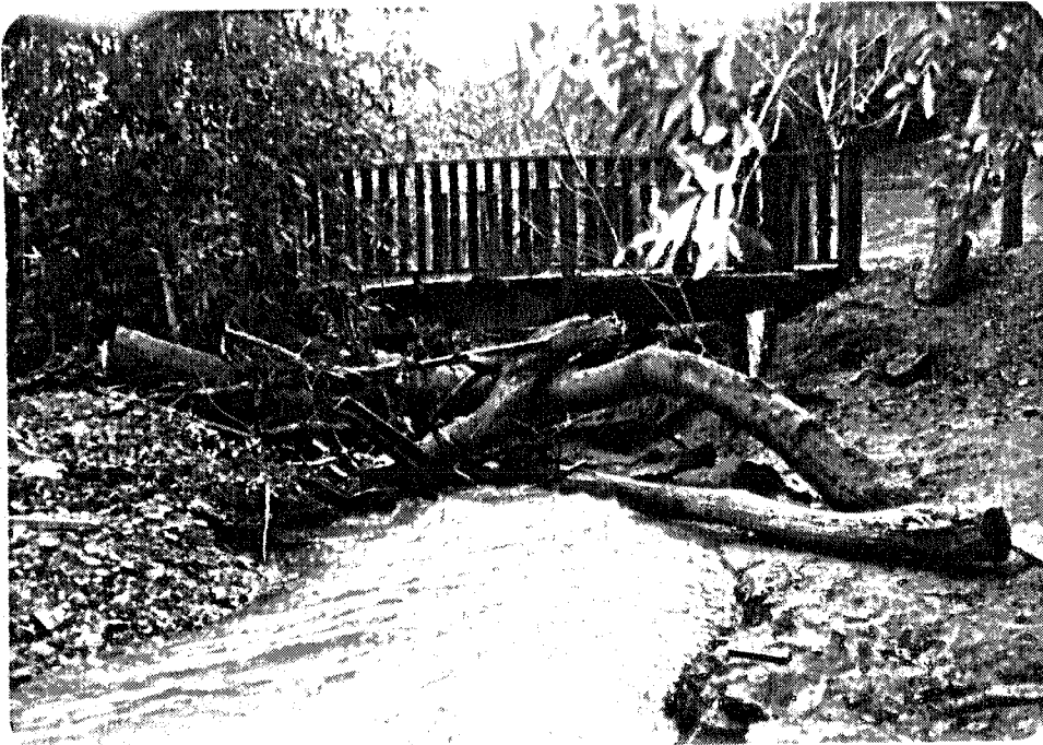
This old structure is showing its age. This is Guadalupe River upstream of Malone Drive. The lining is beginning to fail and erosion is occurring behind the wall.
