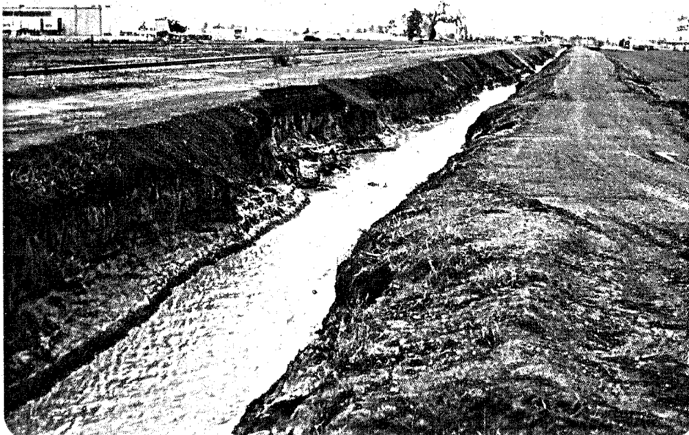
Erosion damage similar to that shown in this photo constituted a good part of the damage imparted by these storms.
